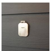
4) Check cover alignment and operation. Adjust friction hinge if peoded
