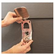
2) Slide the existing cover up to remove. New cover must be installed BEHIND the hydrant faceplate.
