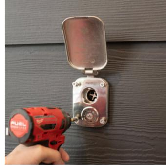
3) Replace mounting screws to secure assembly to wall.
