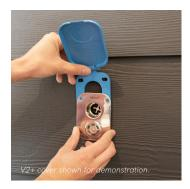
1) Remove existing cover by releasing hydrant mounting screws. There is no need to shut off the water supply. Do not disconnect from plumbing.
