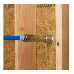
3) Attach to PEX tubing using appropriate tool and expansion ring. Check for leaks and test the hydrant operation.
