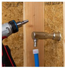
2) Hand tighten new inlet on hydrant body by threading clockwise.
